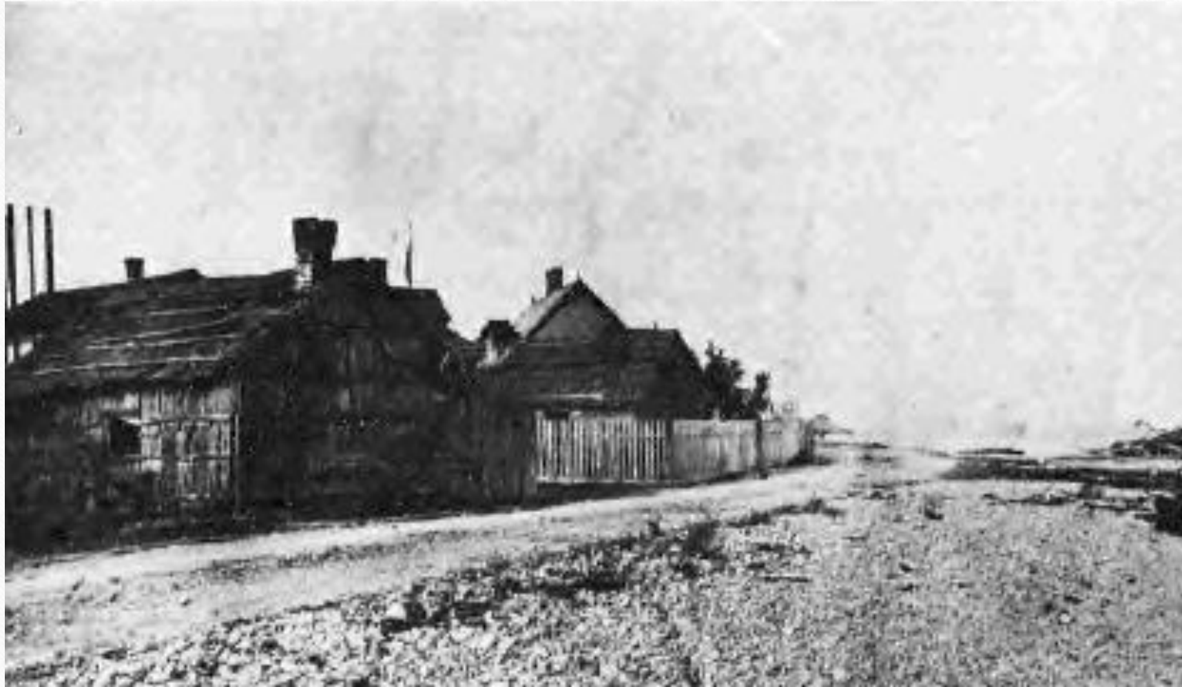
Cadotte Homes made of logs and sided with bark at Biddle Point, Mackinac Island.
